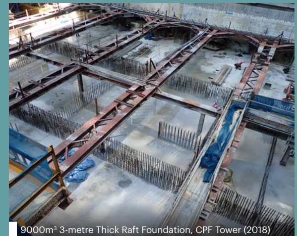
9000m 3 3-metre Thick Raft Foundation, CPF Tower (2018)
